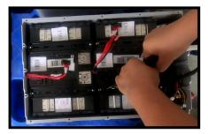
4.3.10 Re-connect the copper bar and battery module's positive and negative cables.
