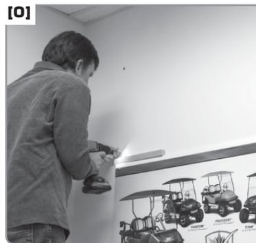
**O]** Remove Header and install Wall Anchors.
