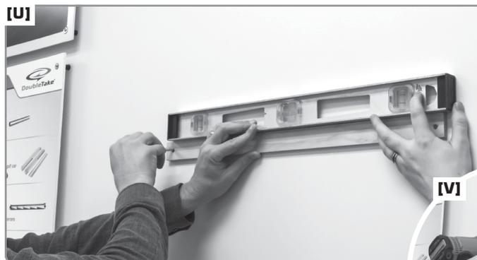
**U]** See the layout reference above for proper spacing. Position the Cushion Hanger Wood, make sure it's level, and mark hole locations.
