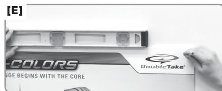
**E]** Level the Panel and mark the opposite top hole. Lower Panel and install EZ Wall Anchor.
