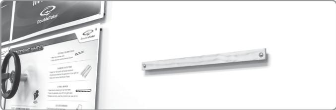
**W]** Mount the Cushion Hanger Wood using provided hardware and 1/2" Black Spacer between wood and wall.
