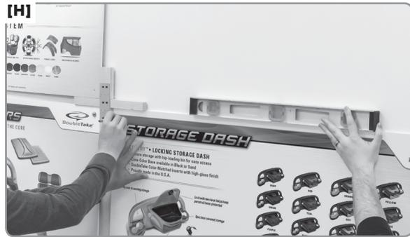
**H) \*\* 2-PERSON JOB\*\*** Using the Install Jig on the right edge, position the next Bottom Panel, make sure it's level, and then mark all 4 mounting locations.
