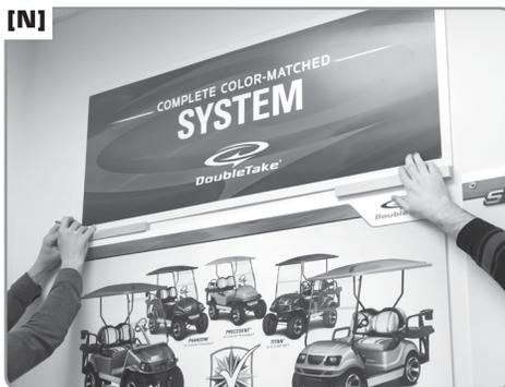
**N]** **\*\* 2-PERSON JOB\*\*** Place the Header onto the 1" tall wood spacers (taken from Jigs in **(K)** above).
