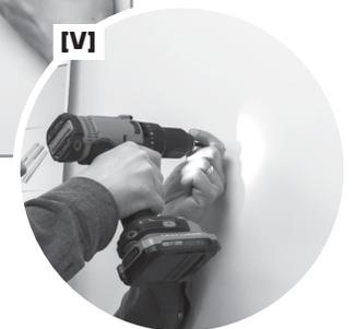
**V]** Install Wall Anchors where marked.
