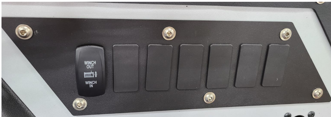
Figure 11: Winch switch Installation
